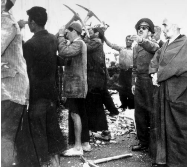
Mullah Falsafi supervising workmen in the act of destroying the dome of the National Bahá'í Center in 1955, Tehran.
